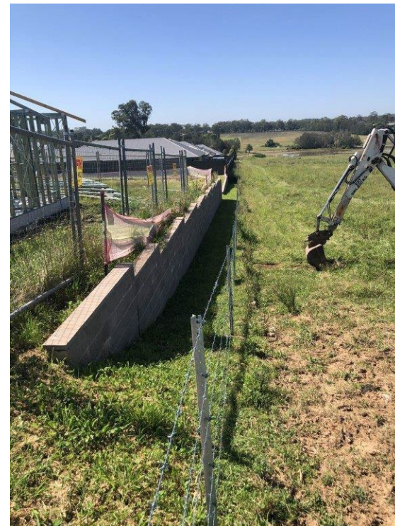
Photo 6: Disused water pipe not located north of dam along eastern boundary – AEC 8
