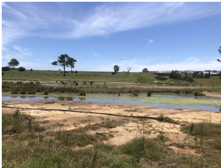
Photo 5: Disused water pipe laying on ground near dam – AEC 8
