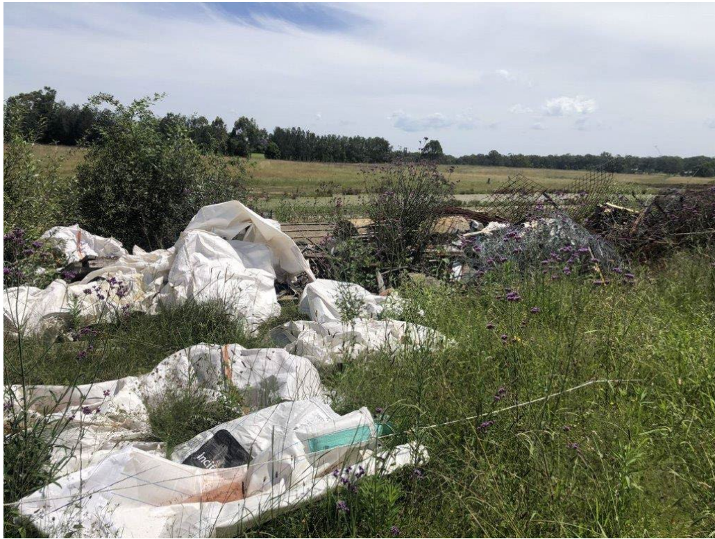
Photo 10: North concrete structure filled with dumped wastes – AEC 12(N)
