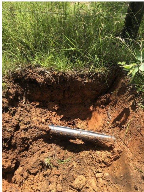
Photo 4: Disused water pipe located along eastern boundary at southern corner – AEC 8
